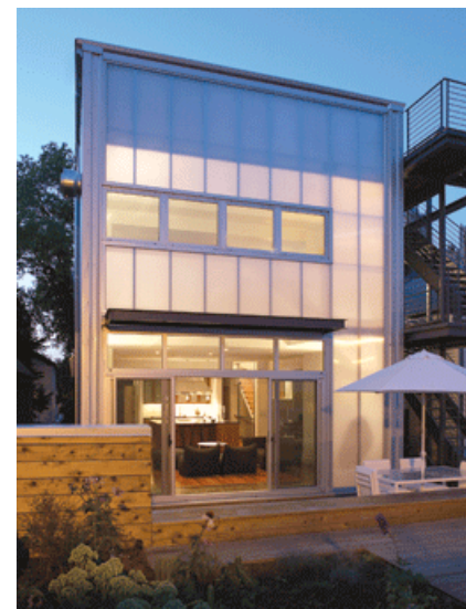
Translucent panels across the rear of the house don't even hint at what the front facade looks like. The house is actually a Victorian three-flat. Photos courtesy of Wilkinson Blender
